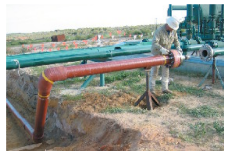
Preparing for hydrotest prior to tie in to facility
