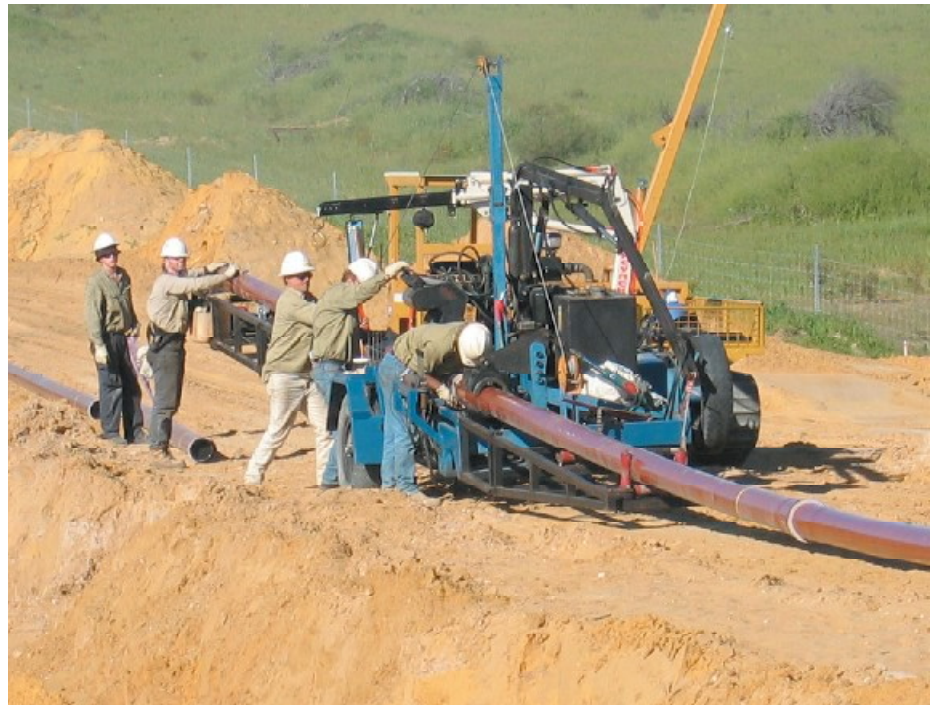
Full work crew for 6" pipe.
