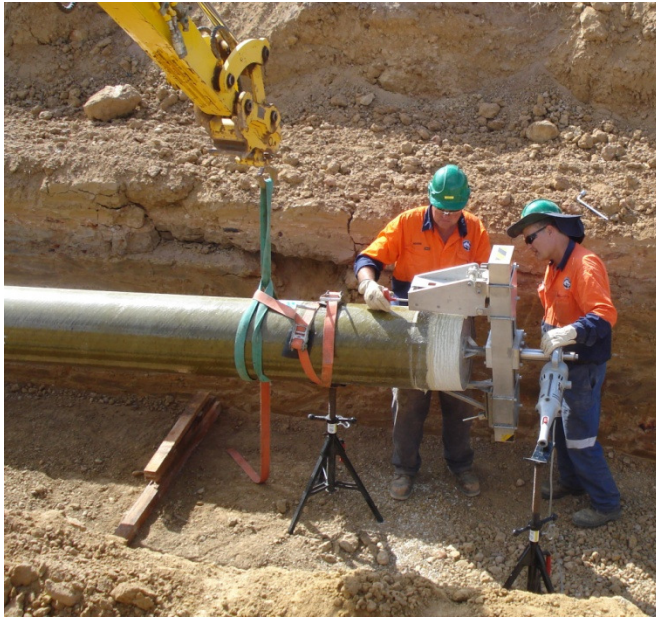
Shaving male spigot for Bell and Spigot pipe joint
