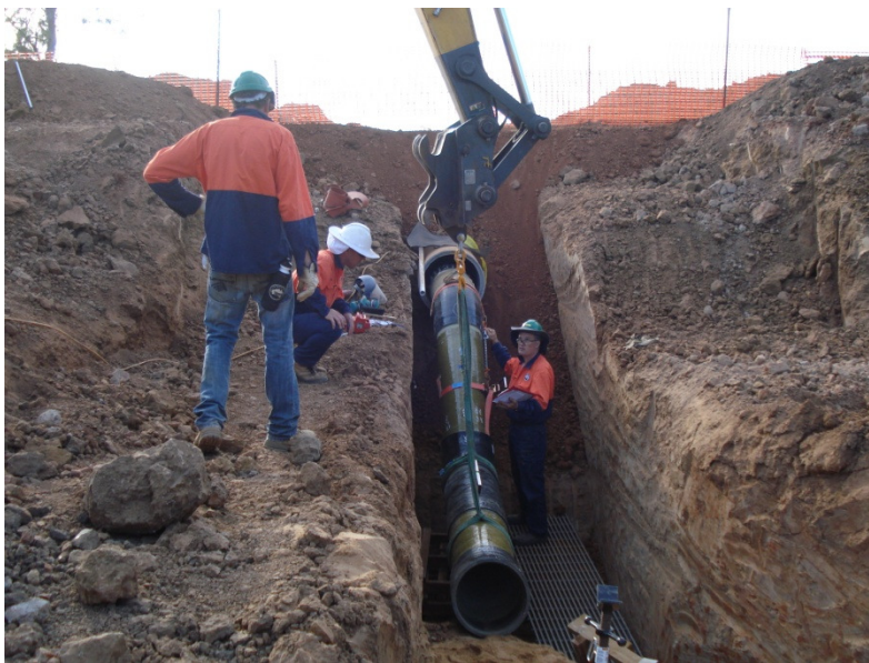
Plant road and drainage channel crossing
